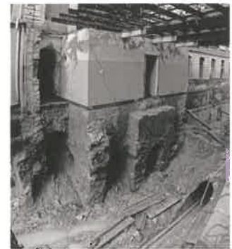
Com a escavação observaram-se os assentamentos bem como a dispersão de águas e esgotos produzidos no subsolo. Todos os trabalhos tiveram acompanhamento arqueológico. (Arquivo VMISA Arquitectos, Janeiro 2009) With the excavation ground cavings as well as water and sewage dispersion produced in the subsoil were observed. All works had archaeological assistance. (VMISA Arquitectos Archives, January 2009)
